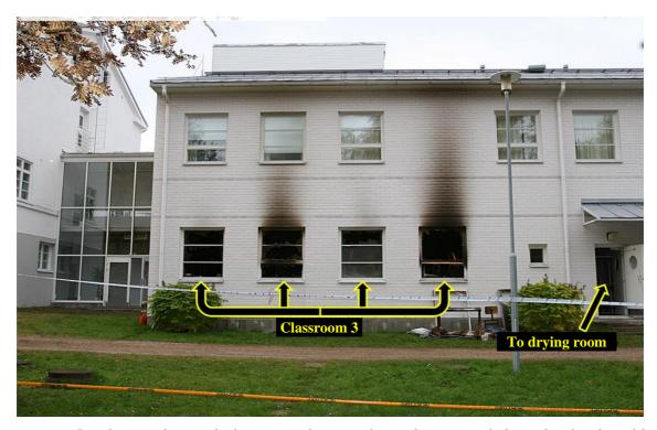
Picture 5. The windows of classroom 3, seen from the rear of the school. The old section and corridor are on the left. The outer walls of the building are made of stone. (Picture from police investigation material)
